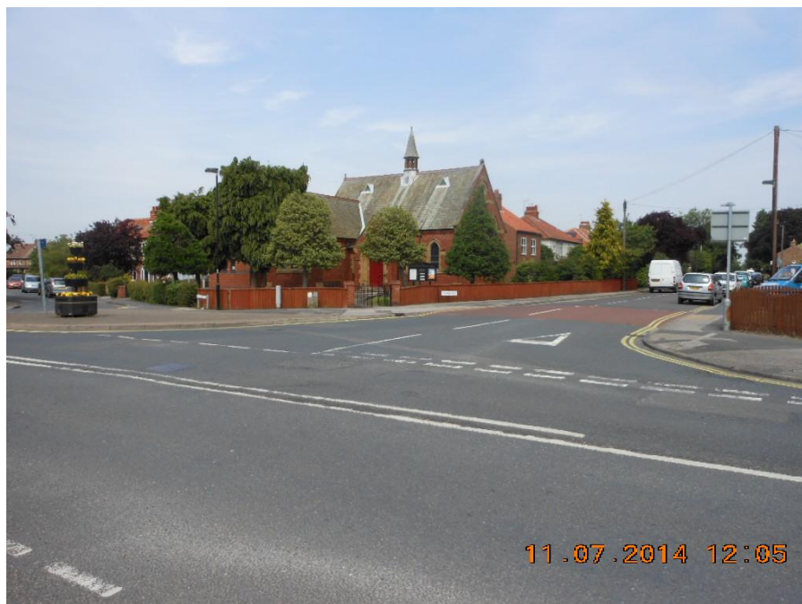
Photograph 01: From the south side of Main Street looking in a north-westerly direction towards the junction of Sim Balk Lane, the speed table crossing point can be seen in red material.
